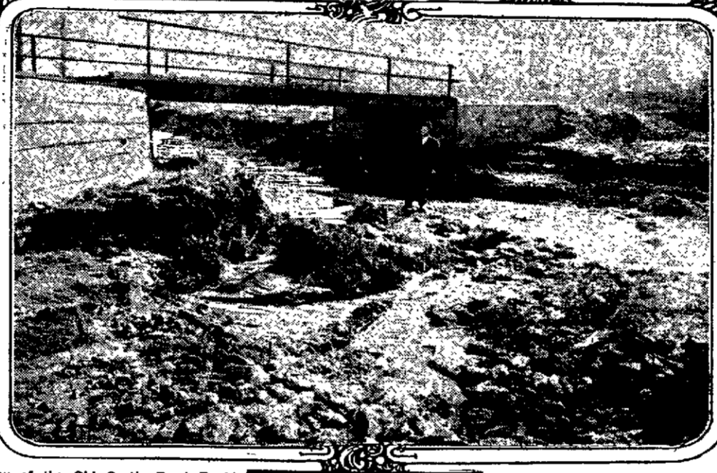
View of the Old Gratis Road Ford Across Jack's Creek, and the New Steel Bridge With Concrete Abutments and Elevated Approach.
