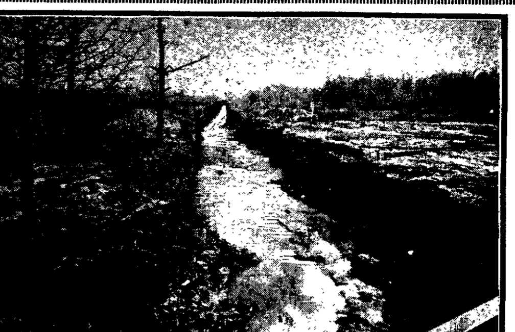
View of Completed Main Ditch on Jack's Creek, Showing How Crooked, Shallow Stream Has Been Straightened, Deepened and Widened.
