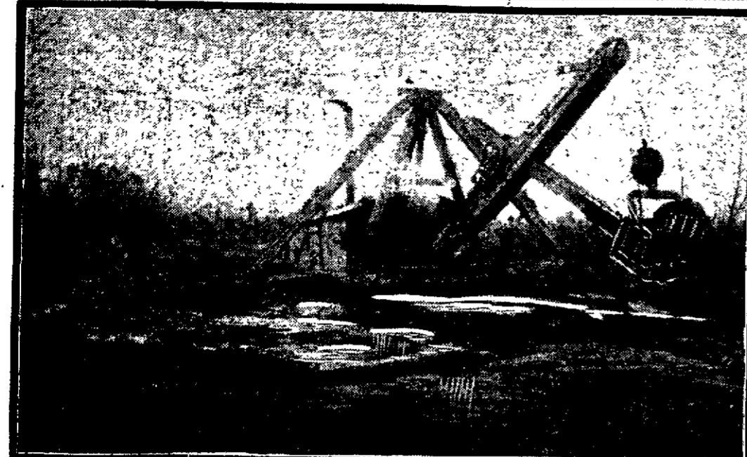
Dredge at Work on Jack's Creek Drainage Project Near Monroe, Ga., With View of Swamp Land Being Reclaimed.
