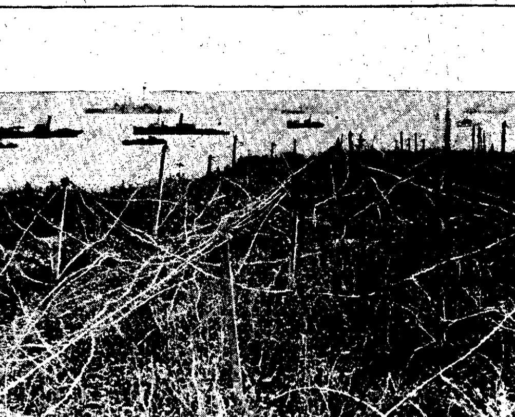
ALLIED SHIPS IN DARDANELLES. BARBED WIRE ENTANGLEMENTS. Some of the barbed wire entanglements near Sedul Bahr are still in position. It will be noticed on the left of the picture that the tops of the supports holding up the barbed wire are serrated so as to add to the formidable nature of the defense. Ships of the allied fleets are seen in the distance.
