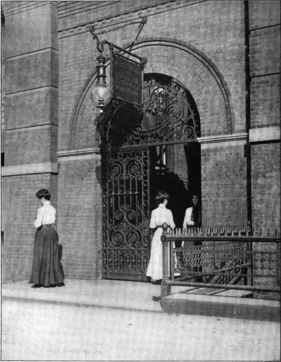
WROUGHT-IRON GATE AT THE ENTRANCE TO THE COURT-YARD.
